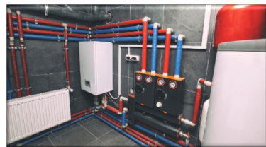
Figure 1: Plumbing System Installation
