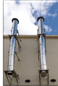
Figure 22: Ventilation Pipes
