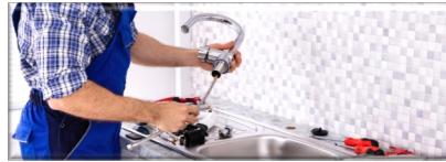
Figure 3: Installation of a Kitchen Sink Faucet
