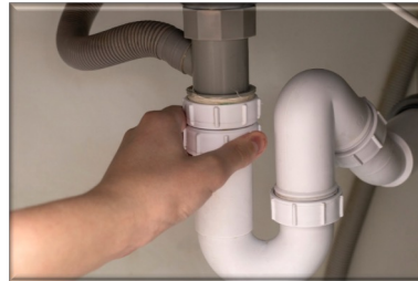
Figure 23: Fixture Traps
