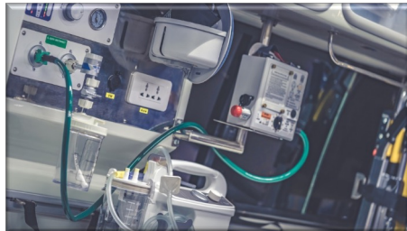
Figure 8: Healthcare Gas Pipe System
